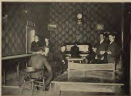
A corner of one of the rooms
